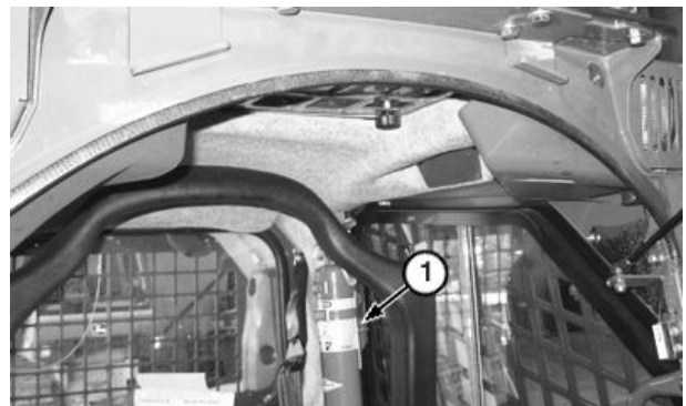
Fire Extinguisher Mounting Location
